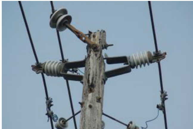
Figure AH-1: Pole Top Deterioration
