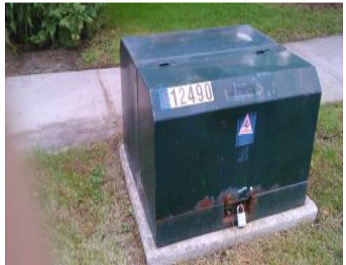
Figure AH-2: Padmount Transformer Deterioration (18 years - 30 years)
