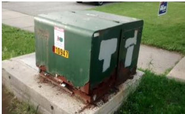
Figure AH-2: Padmount Transformer Deterioration (18 years - 30 years)
